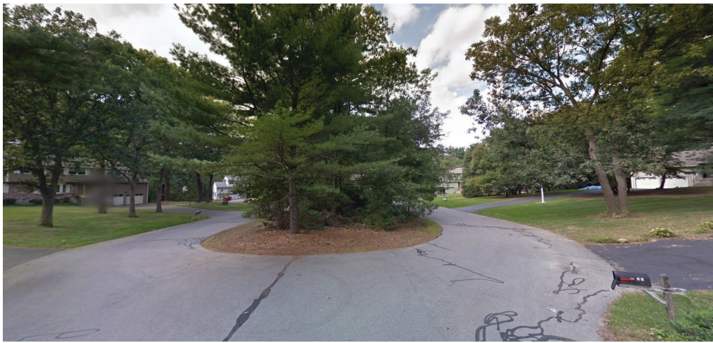
The center islands can be landscaped heavily and built as soft infrastructure to capture runoff and create shade/calm traffic
