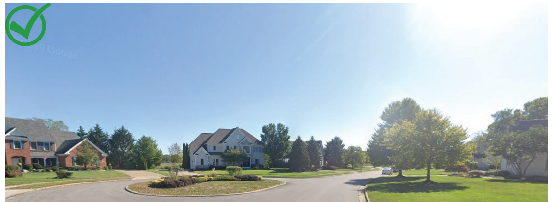
Utilize eyebrow style medians to calm traffic, create greater spacing for homes off of the main roadway and preserve greenspaces
