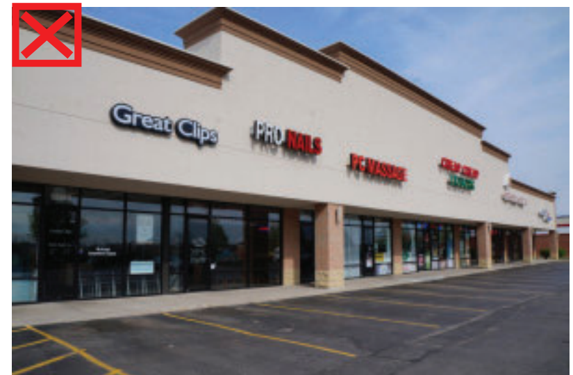
Avoid long expanses of uninterrupted and unvaried facades fronting on parking lots/drive aisles
