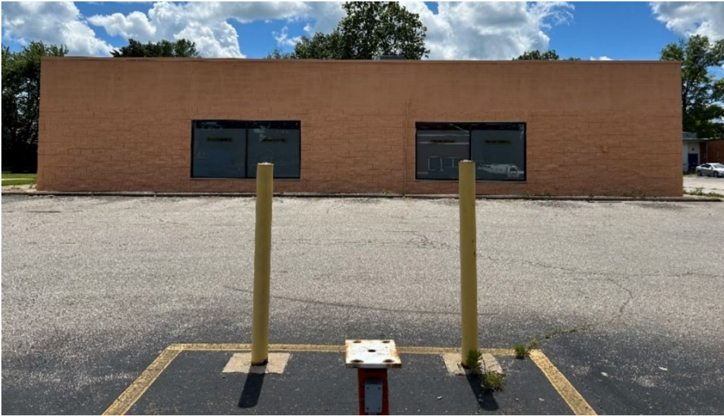
Existing (view from SR 125 – Main)
