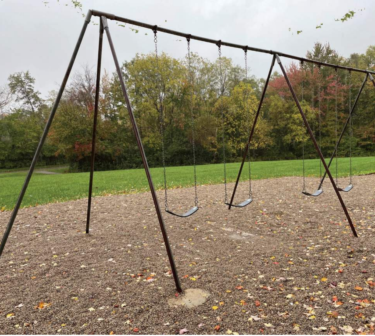
F. EXISTING SWING SET WITH EXPOSED CONCRETE FOUNDATIONS
