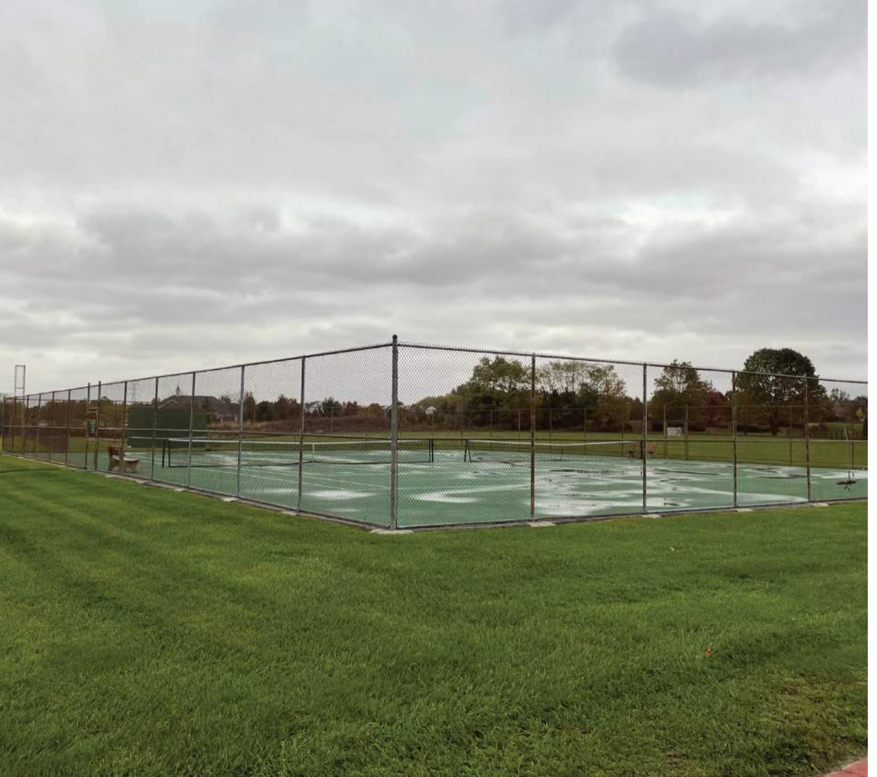
L. EXISTING TENNIS COURTS
