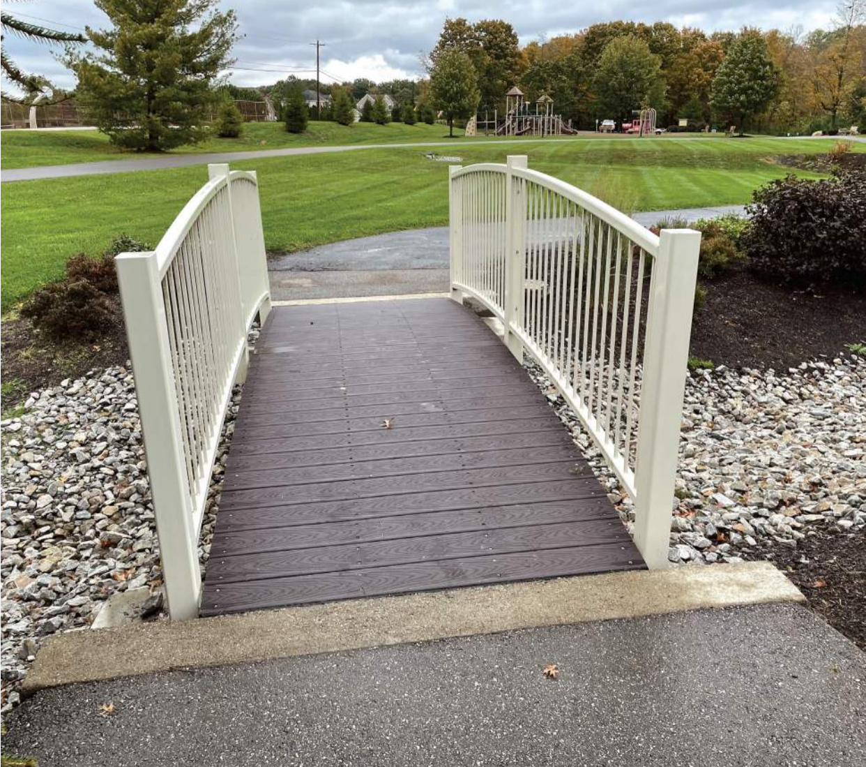
F. EXISTING PEDESTRIAN BRIDGE
