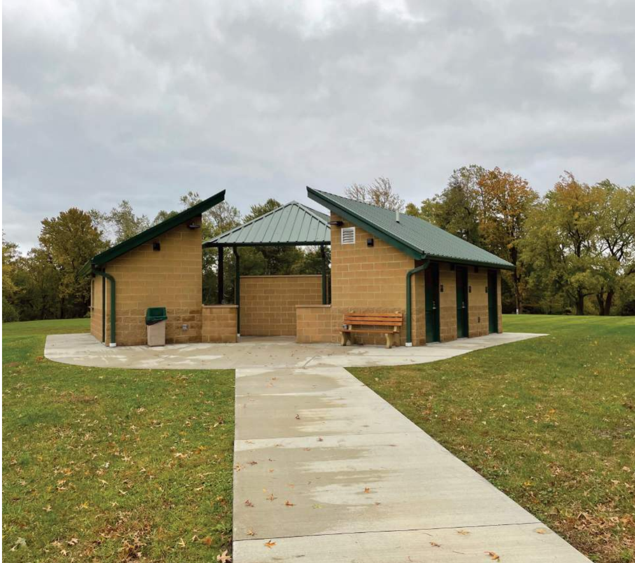
H. EXISTING RESTROOM AND STAGE FACILITY
