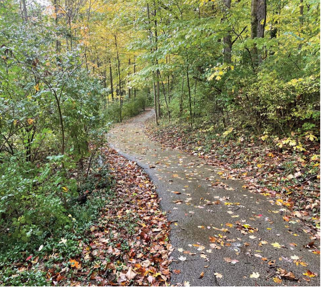
O. EXISTING ASPHALT TRAIL
