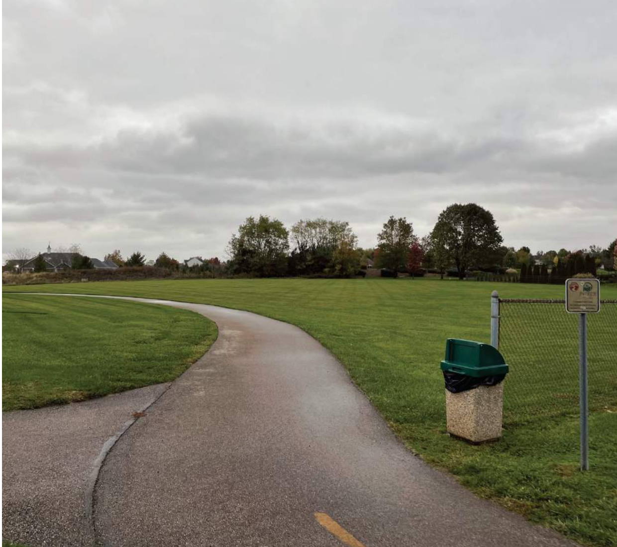
M. EXISTING ASPHALT TRAIL
