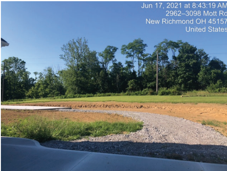
View to the South
