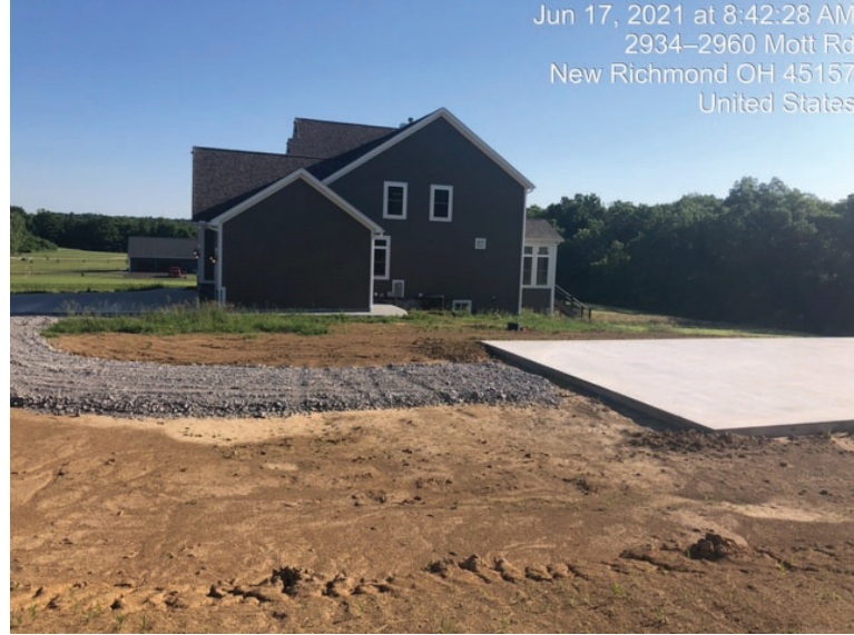
View to the North
