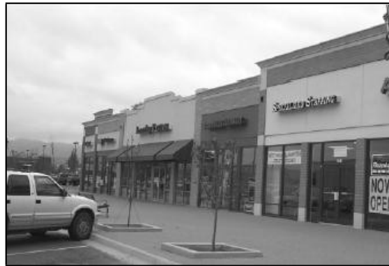
Figure 9-3: Illustration of roofline changes that are aligned with façade offset and changes.
