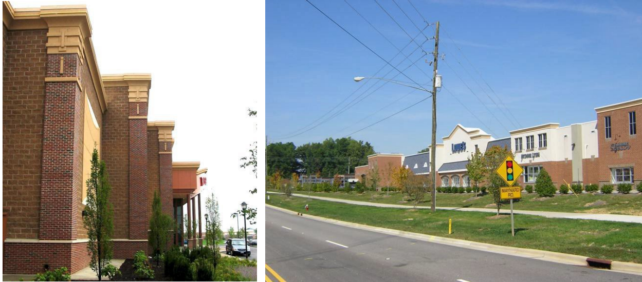
Figure 9-1: The buildings in the above images contain pilasters, cornices, and a series of façade setbacks (recesses) to visually break up the appearance of large façades.
