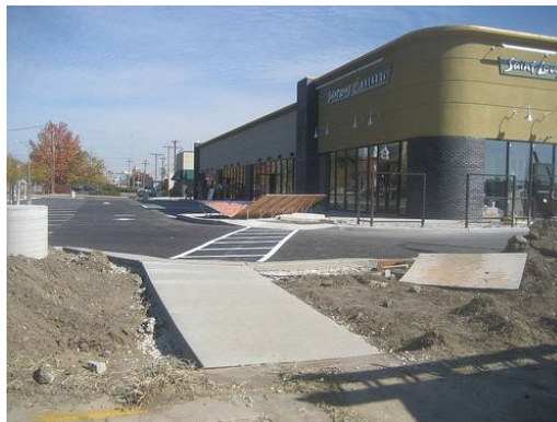
Figure 11-2: This image illustrates a sidewalk connection between a building and a public sidewalk in the right-of-way. This connection includes both a separate sidewalk (foreground) and a connection delineated through a painted line (background).
