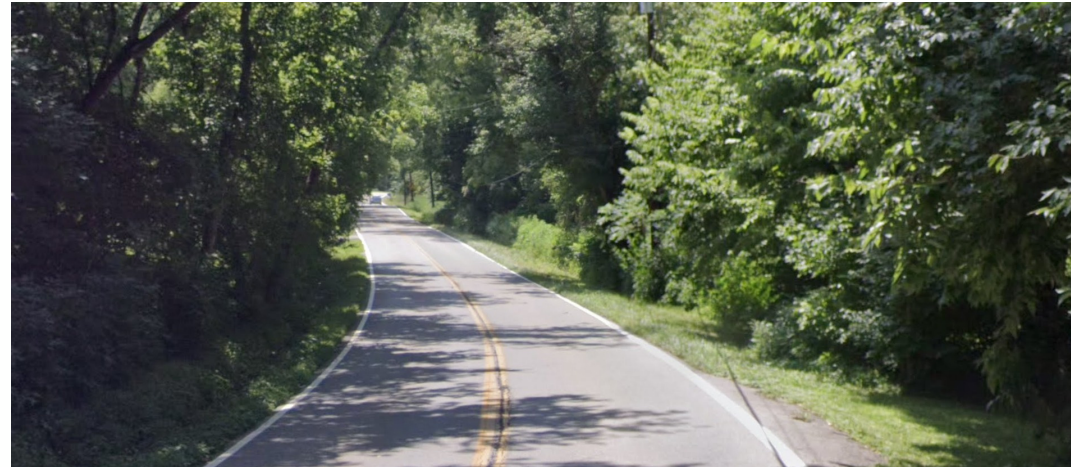
Ninemile Road is an example of a rural route with some geometric constraints
