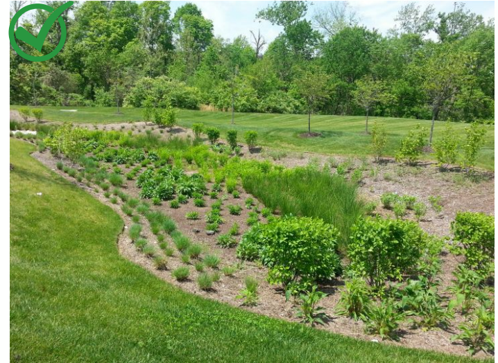
Bioretention areas can be used to reduce stormwater runoff, reduce the need for large stormwater ponds and provide an amenity
