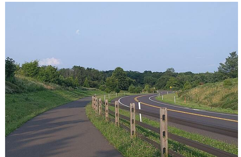
202 Parkway Trail provides a sample illustration of trail, fencing and distance from the roadway
